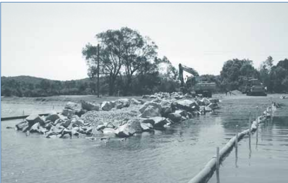
Cockle Creek groyne construction
