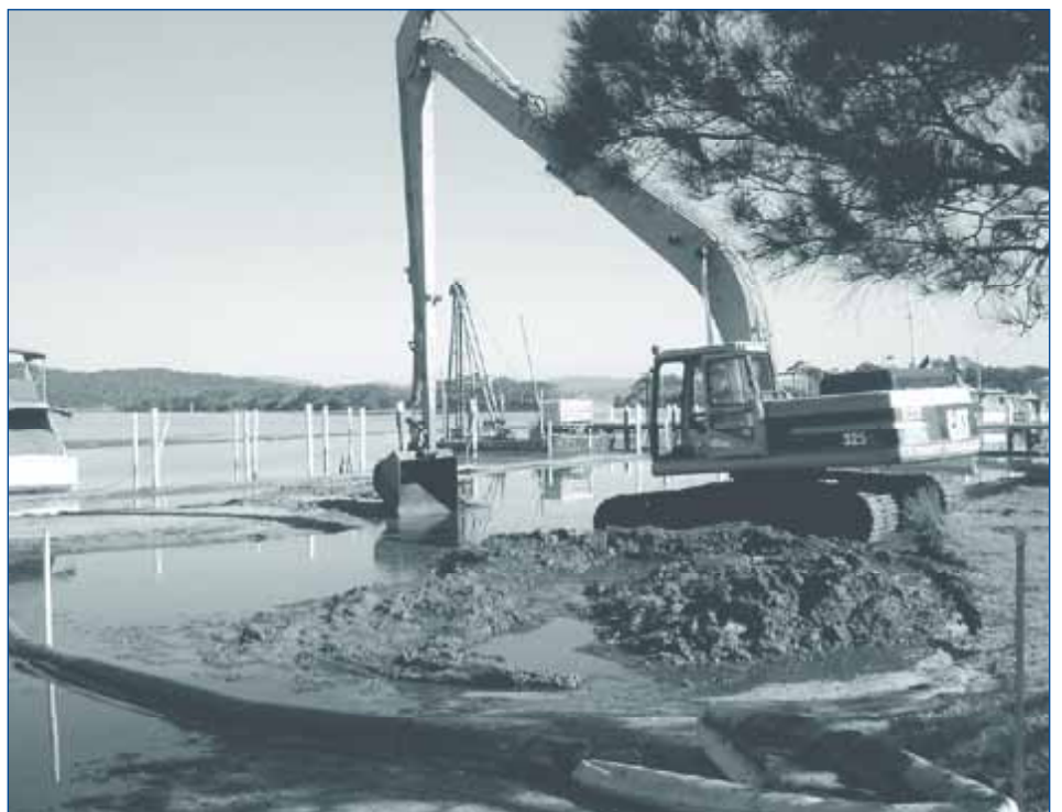
Swansea Flats, nearshore organic sediment removal and foreshore rehabilitation works.
