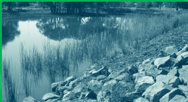
Constructed wetland at William St, Cardiff
