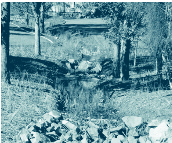
Vegetated riffle ponds replace concrete drain at Gatts Farm Reserve, Valentine.
