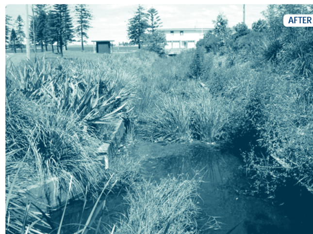
Vegetated concrete channel at Speers Point
