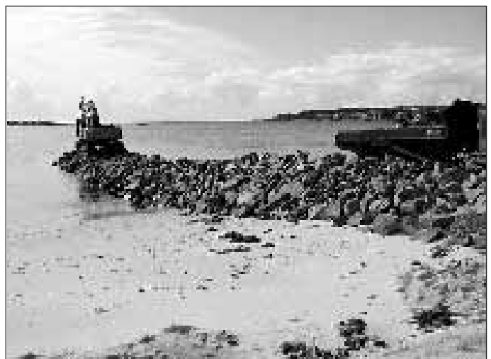
Rock groyne construction for stabilisation of Salts Bay
