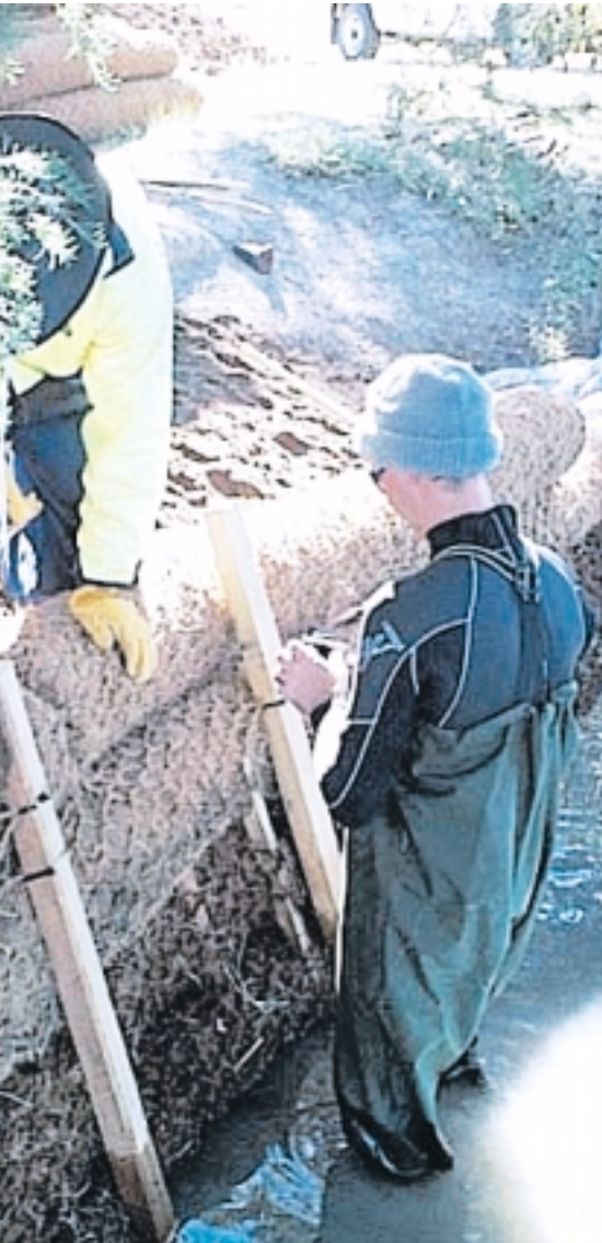
Creek stabilisation works
