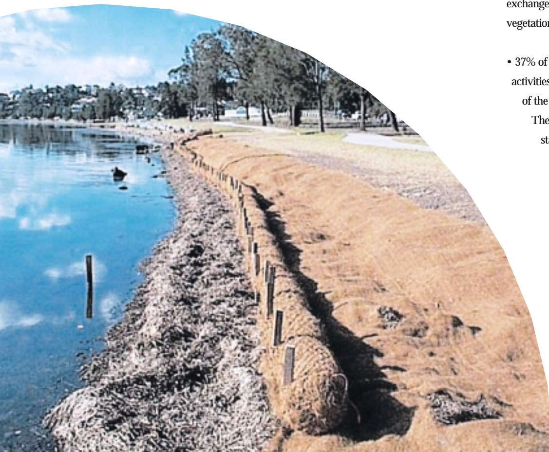
Temporary coconut fibre protection for proposed foreshore planting
