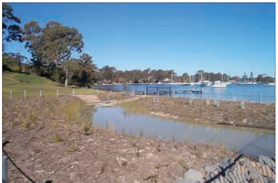
Constructed Wetland Lake Street, Bolton Point
