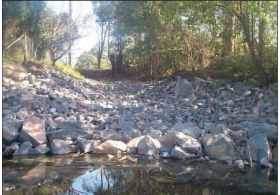
Flaggy Creek stabilisation works
