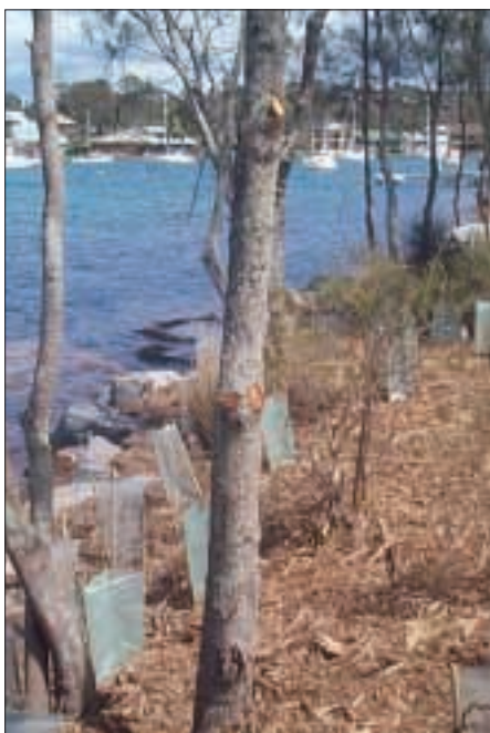
Balmoral Foreshore Reserve Stabilisation Works
