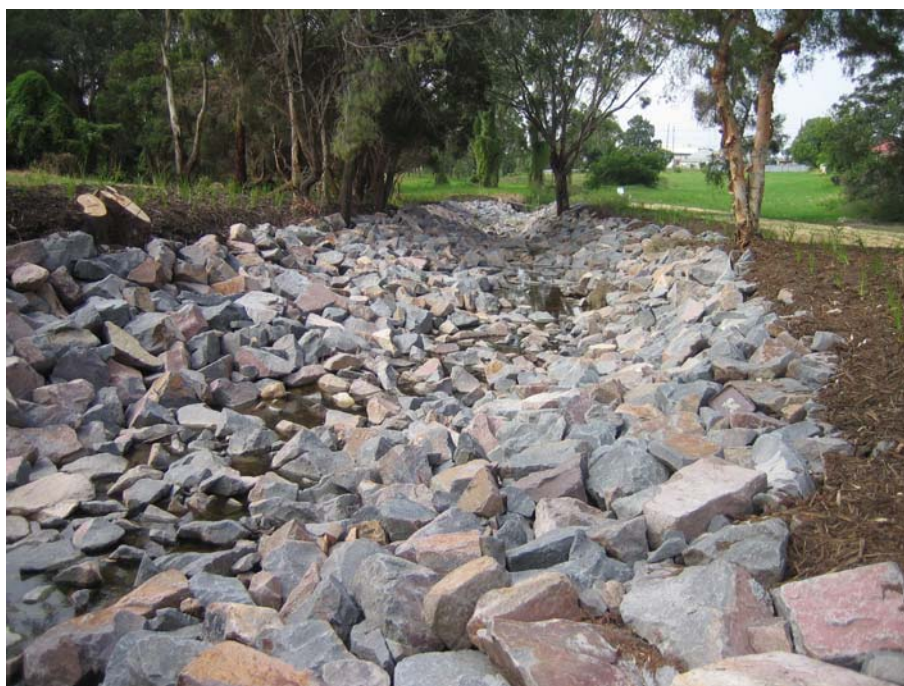
Figure 3 Erosion control works and riffle pools sequences, Edgeworth.
